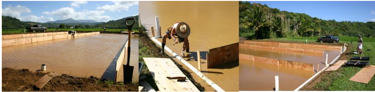
Figure 2. Construction activities associated with the implementation of experimental plots at select Hanalei taro farms.
